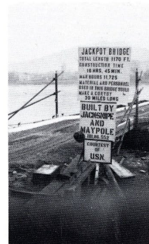
JACKPOT BRIDGE Total length: 1170 ft Construction time: 16 hrs 45 mins Man hours: 11725 Materials and personnel used in this bridge would make a convoy 30 miles long. Built by Jacksnipe and Maypole 181, 86, 552 Courtesy of U.S.N.
