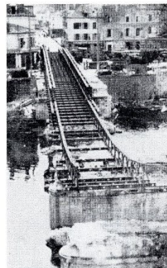
Building Bailey Bridge over the Seine Melun, Aug. 28 - Sept. 2, 1944 (Also known as the "Dinah Shore Bridge")
